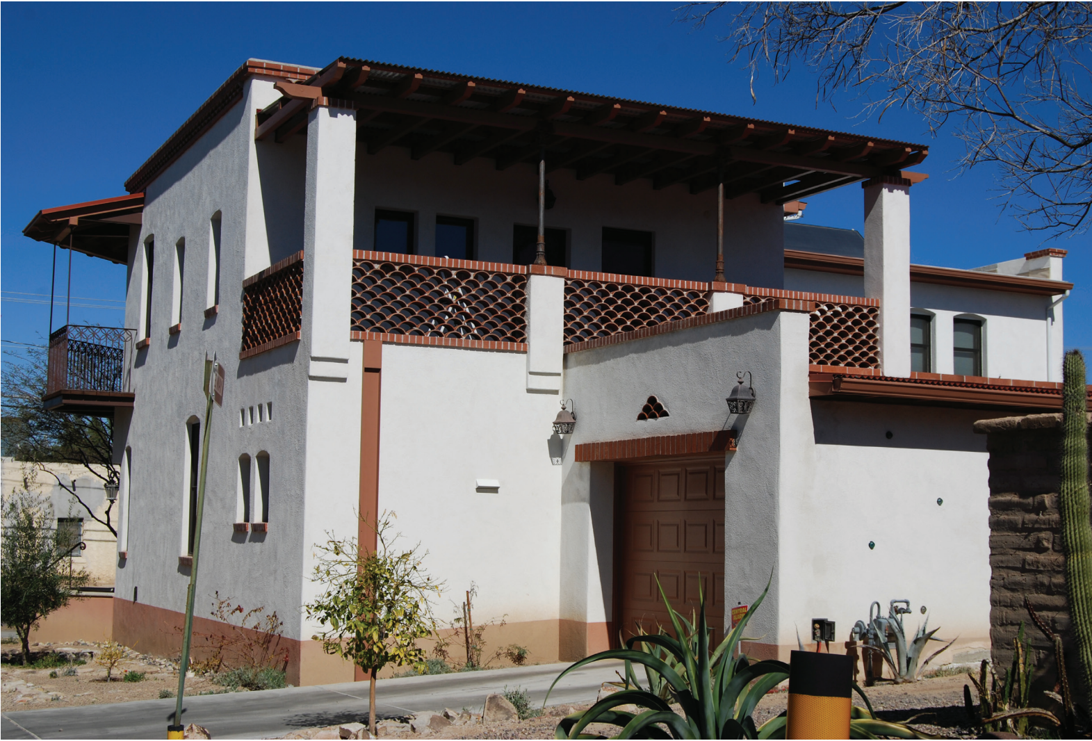
SPANISH COLONIAL REVIVAL This style, which arose in the 20th century, featured additions of smooth stucco walls, low-pitched clay tile, flat roofs, decorative wrought iron trim and small porches or balconies.
